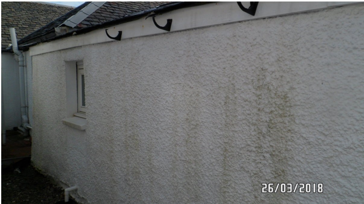
Rear elevation showing obscure glazed white timber window, method of opening unclear.
