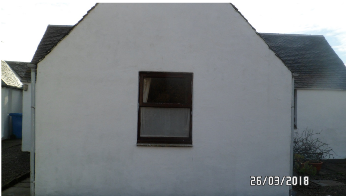
Close up of brown painted timber top hung window to front elevation
