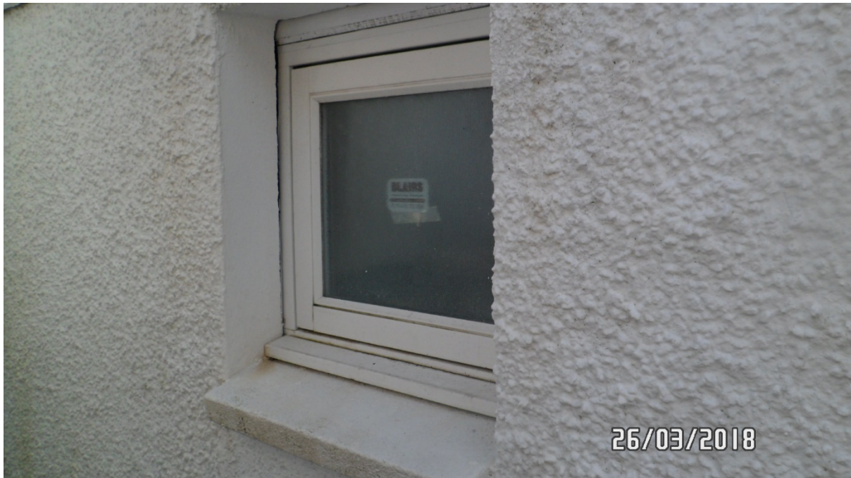
Close up of window to obscure glazed white timber window to rear elevation of single storey projection
