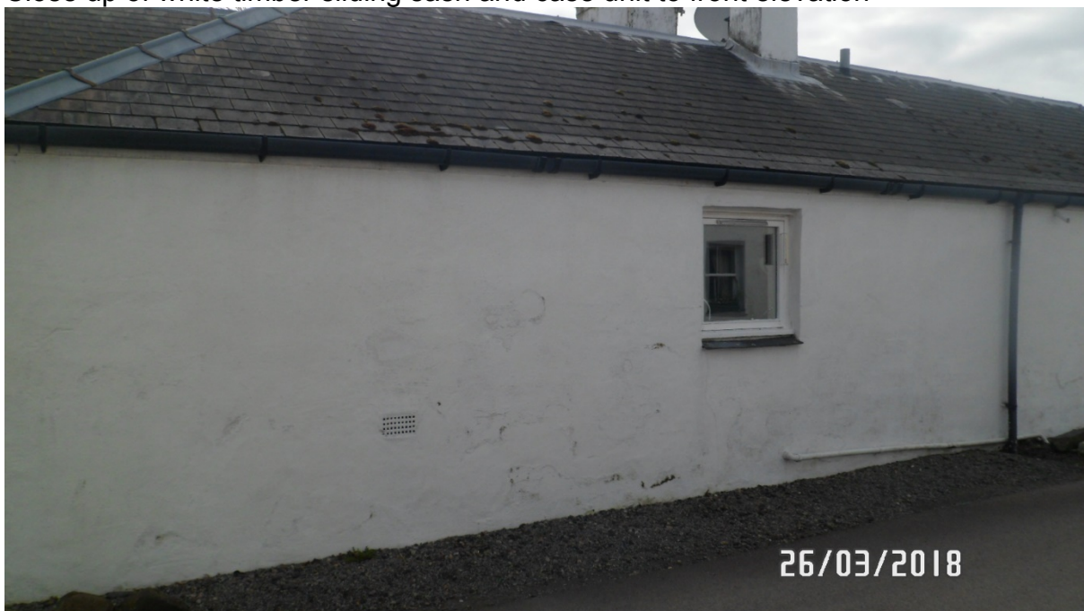
Rear elevation showing 1 no. white painted timber side opening unit
