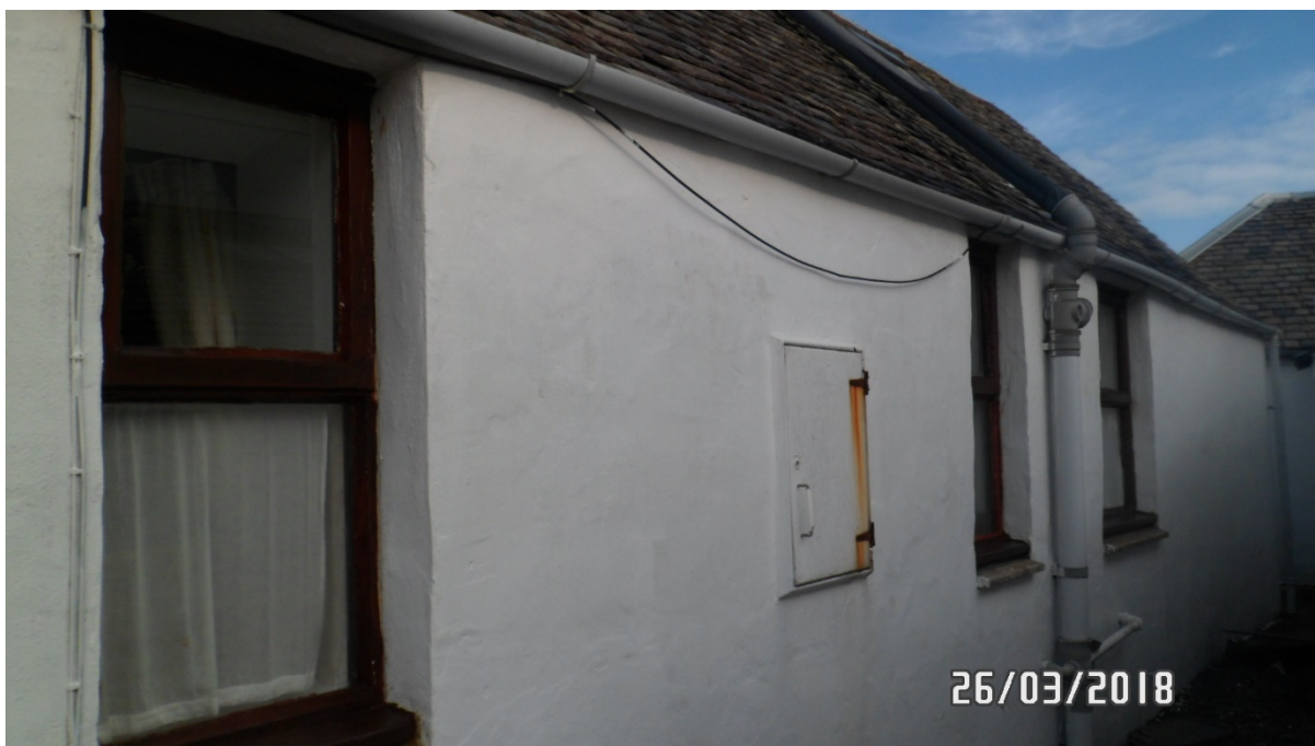
Rear elevation showing 3 no brown timber painted top hung windows
