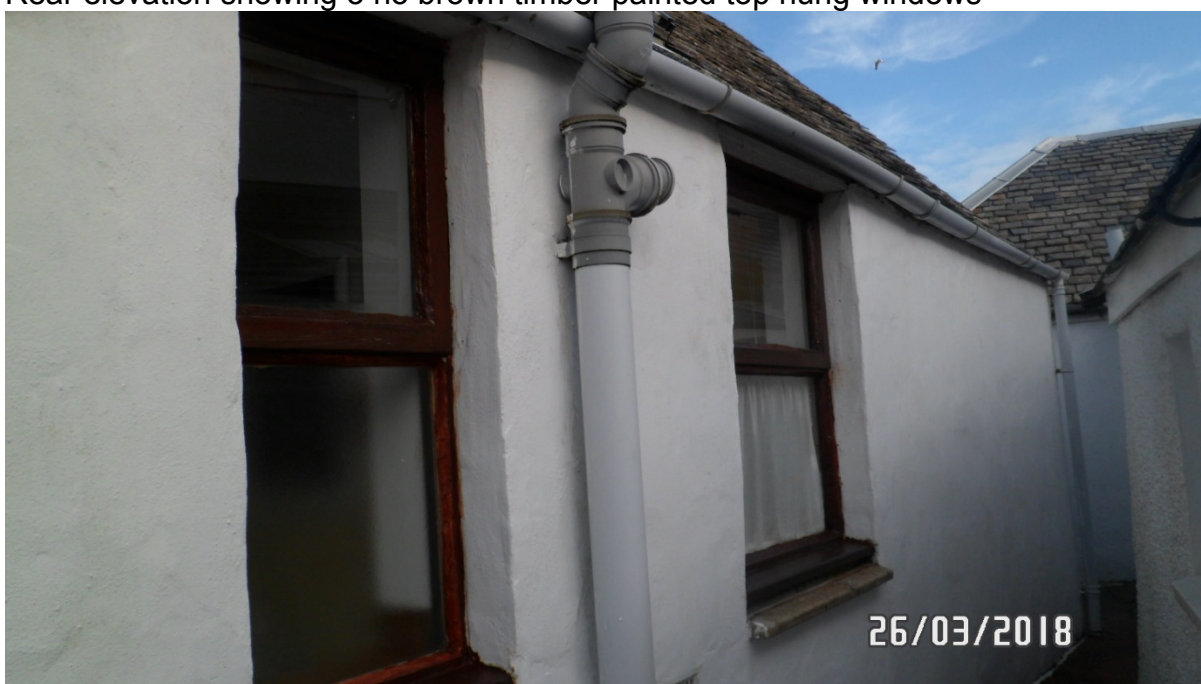
Close up of windows to rear elevation showing brown timber painted top hung windows
