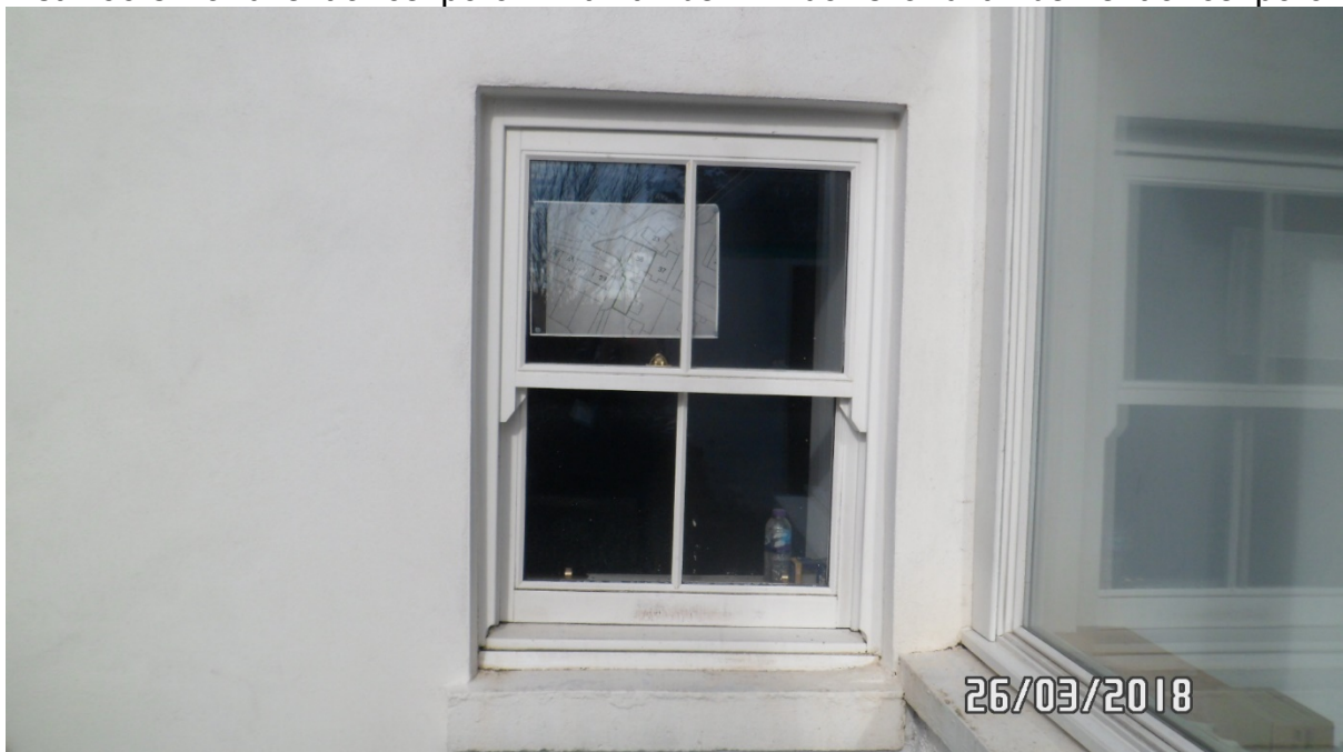
Close up of ground floor white timber sliding sash and case window to left of entrance porch
