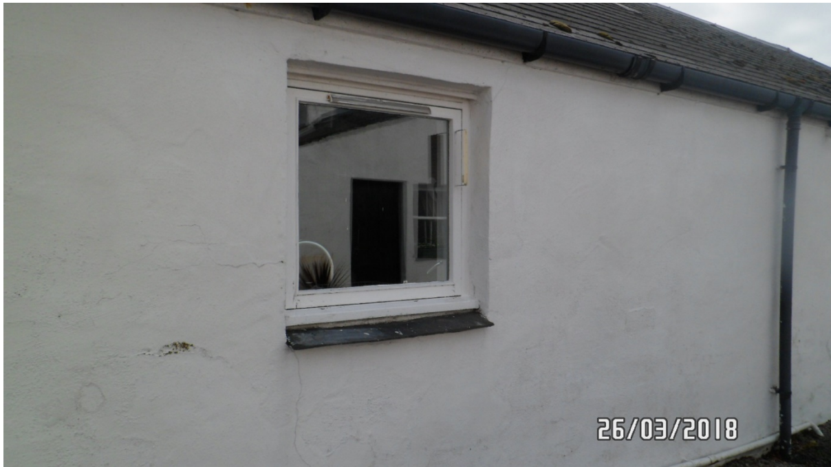
Close up showing white painted timber side opening unit to rear elevation
