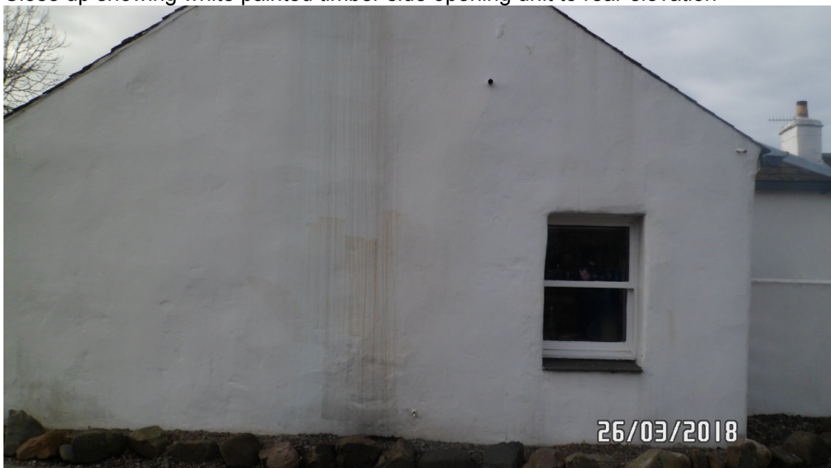
Side elevation showing white painted timber sliding sash and case window
